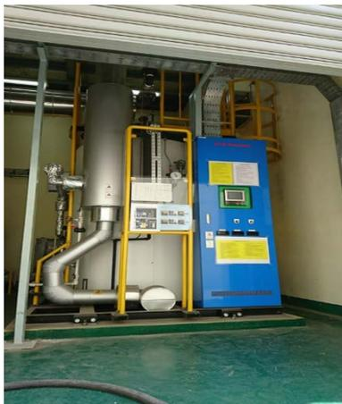
**Gambar 8.16.** *Proyek Introduction of High Efficiency Once-through Boiler System in Film Factory.*
