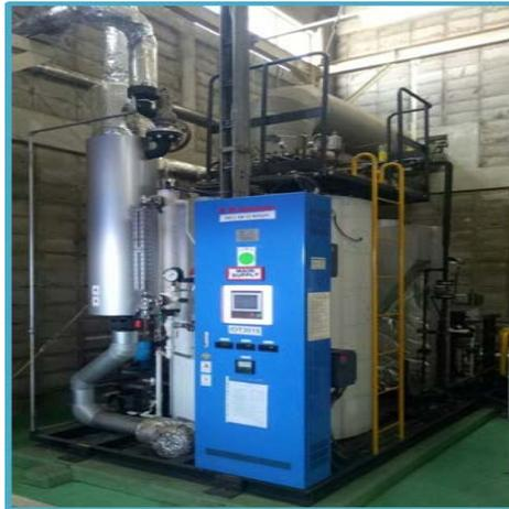
**Gambar 8.15.** *Proyek Introduction of High Efficiency Once-through Boiler System and RO Pure Water System in Golf Ball Factory.*
