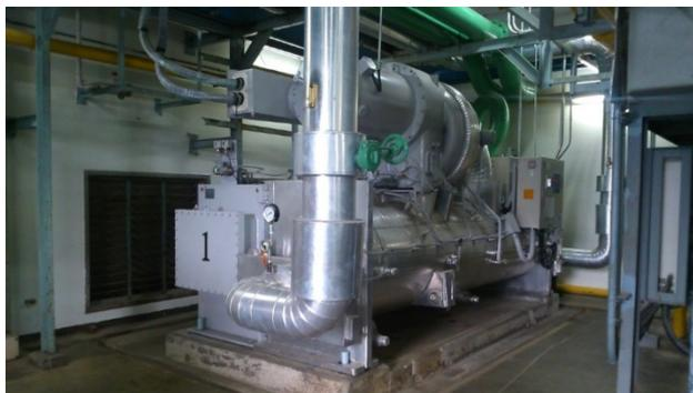
**Gambar 8.10.** Proyek Energy Saving for Textile Factory Facility Cooling by High Efficiency Centrifugal Chiller.
